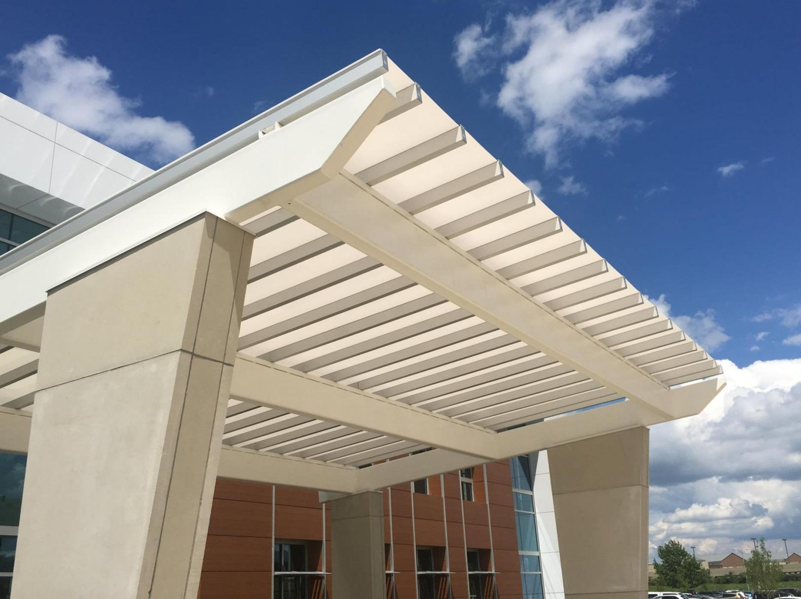
The canopy, from Duo-Gard's award-winning Sleekline Systems, measures 30'6" x 26' and features 1/4" panels of white monolithic polycarbonate sheet, framed in clear anodized aluminum. The choice of this translucent glazing material was the design team's solution to the owner's desire for "openness that complemented the glass in the building's renovation," according to Henderson. She adds that the diffused light the canopy provides contributes to a warm, contemporary aesthetic.
